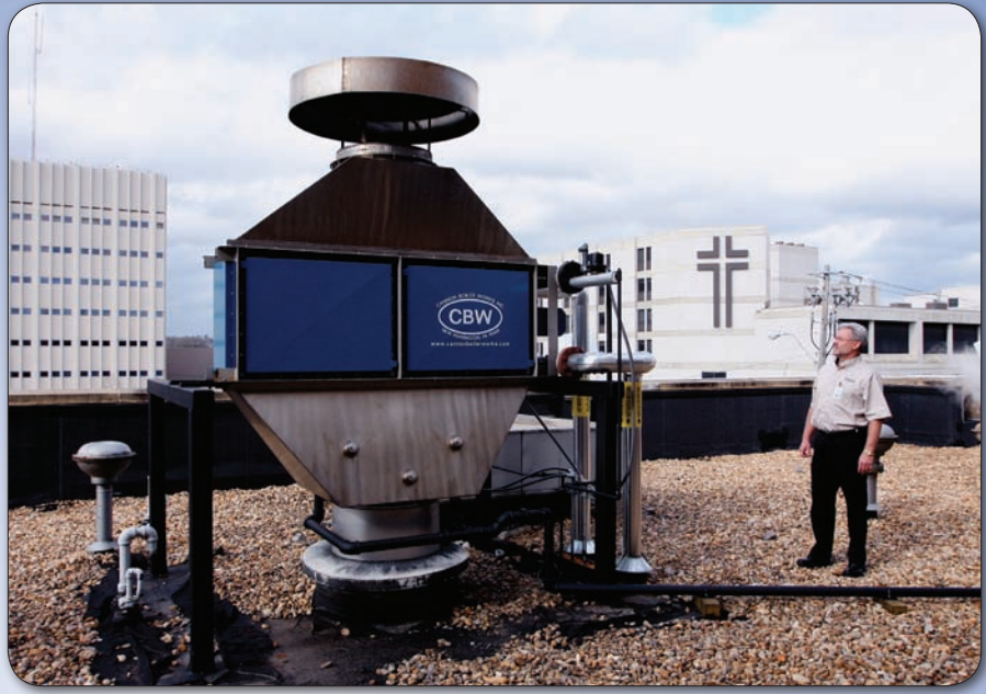
A PLC-based boiler and combustion controls (left) have been retrofitted to the existing boiler. A stack mounted economizer (right) represents technology that works to reduce energy usage and environmental impact.
