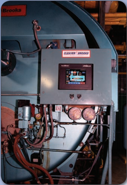
A PLC-based boiler and combustion controls (left) have been retrofitted to the existing boiler. A stack mounted economizer (right) represents technology that works to reduce energy usage and environmental impact.
